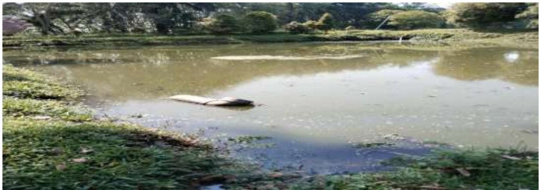
Gambar 1.8 bak penampungan aerob III
